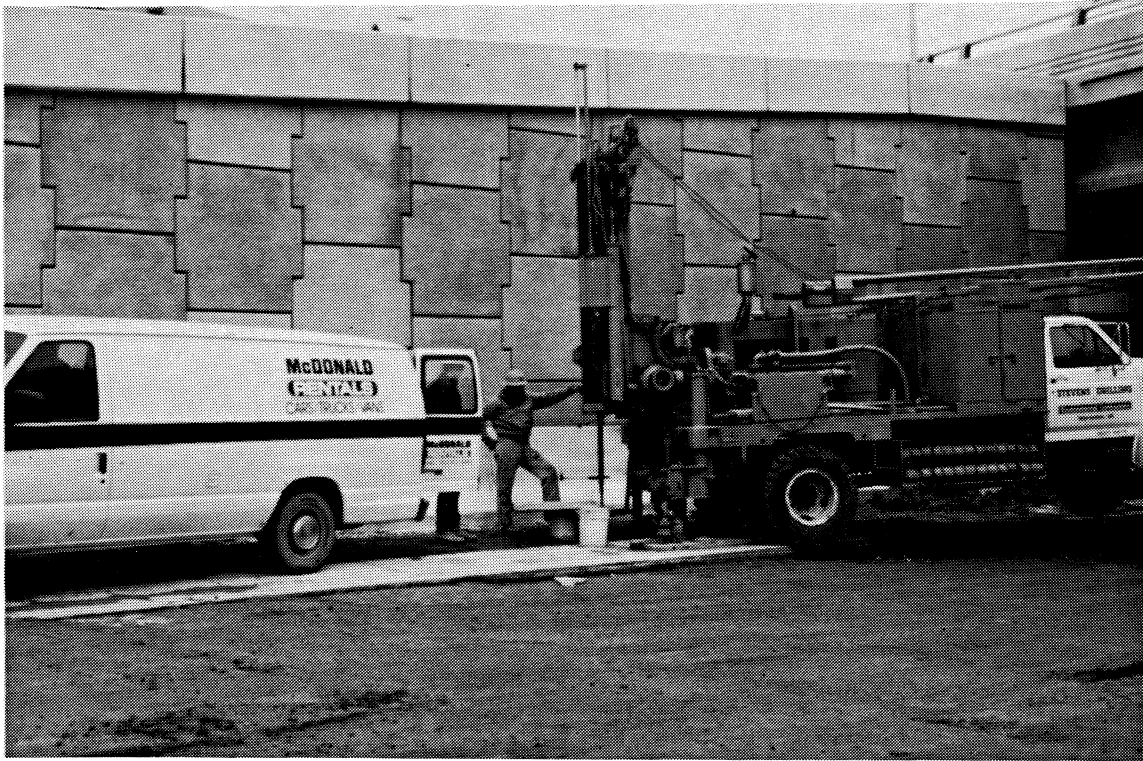
Figure 4.2. Piezocone Testing Operations at Port Huron, Michigan.
