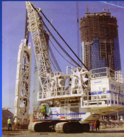
View of Construction Operations
