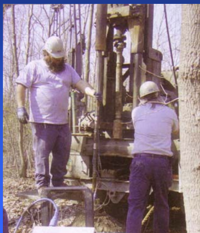
View of Geotech Site Investigation
